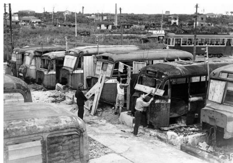
Disabled buses that have littered the streets of Tokyo are used to help relieve the acute housing shortage in the Japanese capital on October 2, 1946. Homeless Japanese who hauled the buses into a vacant lot are converting them into homes for their families. (AP Photo/Charles Gorry)
